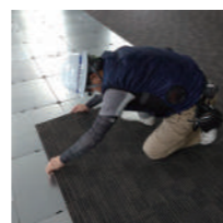
Carpet tile installation
