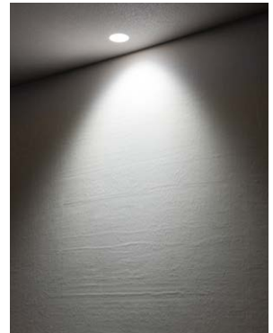
Examples of Adhesive Gaps and Streaks
